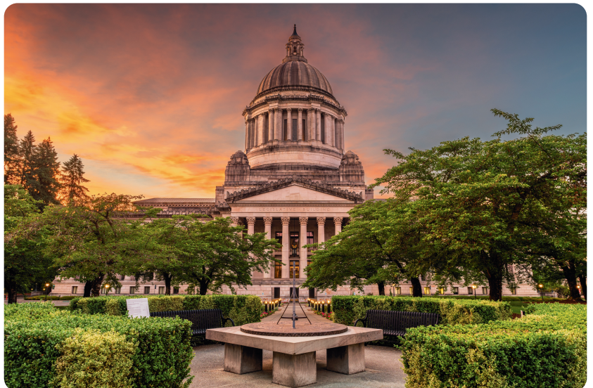
State Capitol Building, Olympia, Washington
